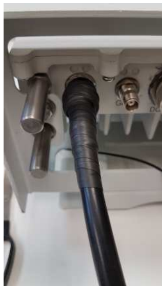
Figure 2-2: Cable Weatherproofed with Self-Amalgamating Tape
