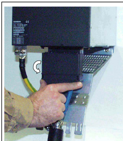
Close the cover of the terminal strip.
